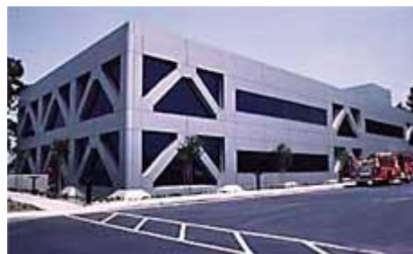
Figure 13 - Los Angeles Fire Department Control Facility
