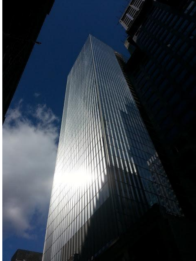
Figure 7 - 250 West 55th Street Building
